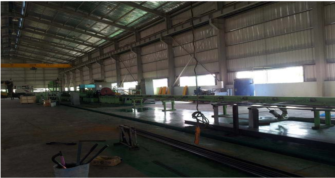
Cambodia Factory Inside
