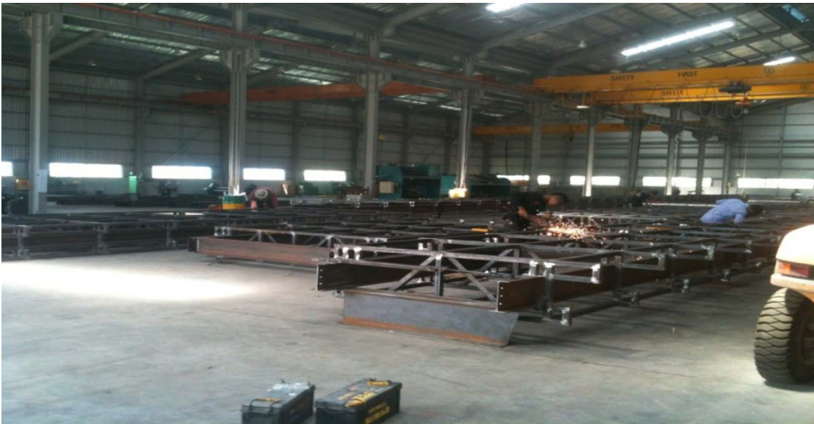
Cambodia Factory Inside
