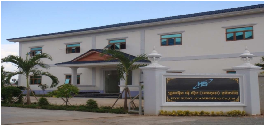
Cambodia Office and Factory
