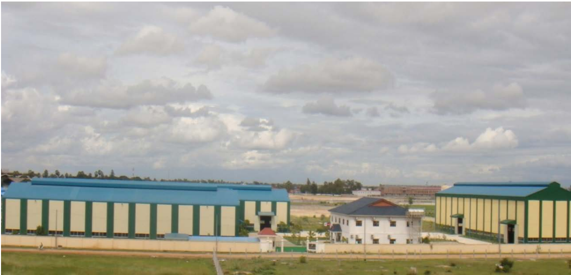
Cambodia Office and Factory
